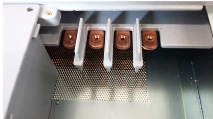
Fig. 11 – Connection for Element for Auxiliary Switchboard derivation ex DY3200 - Annex 3
